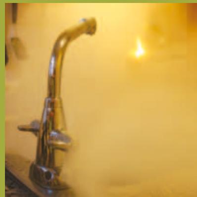
The system uses a high-pressure pump to generate a fine water mist from nozzles mounted under a kitchen monobloc tap, on a work surface or in a wall. Versions are available for protecting living rooms, kitchens, and open or semi-open kitchen/diners.
