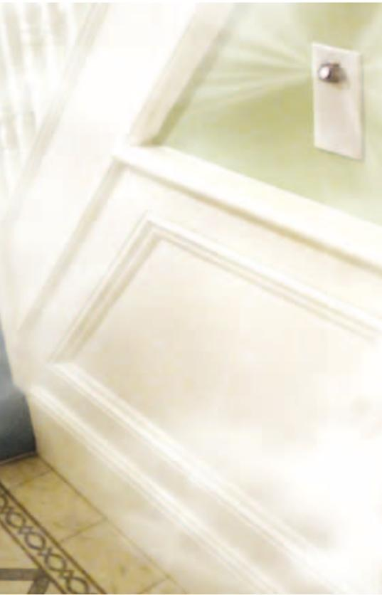
water mist devices have now emerged on the market, which can be fitted without compromising building layout or aesthetics and with minimal disruption.
