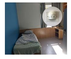
A custom pre-engineered Automist Fixed system was the ideal solution for 14 rooms in Prospect Park Mental Health Hospital. It featured an antiligature head and a key switch control outside each room which staff could operate. The installation was completed in one day to minimise patient disruption.
