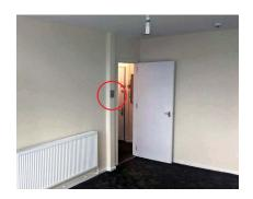
Automist can be installed on a flat-by-flat basis, to prioritise vulnerable individuals identified by a fire risk assessment. It is often more cost effective to retrofit than sprinklers because it uses the existing water supply in the dwelling. Automist provides industry standard (BS 8458) fire performance. The installation was well received by residents because of its discrete design.
