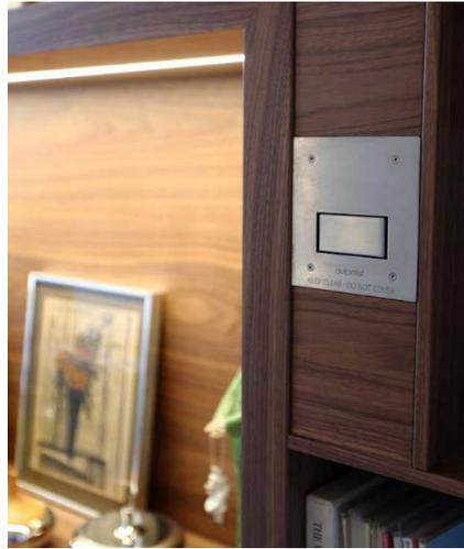
Figure 20: Preferred position built into a cupboard or joinery
