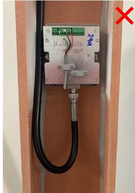
Figure 54: At risk trunking installation with hose bending
