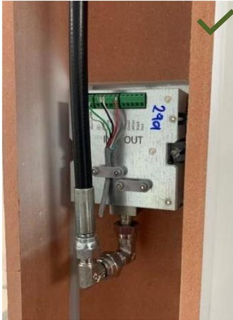
Figure 53: Correct trunking installation with double elbows
