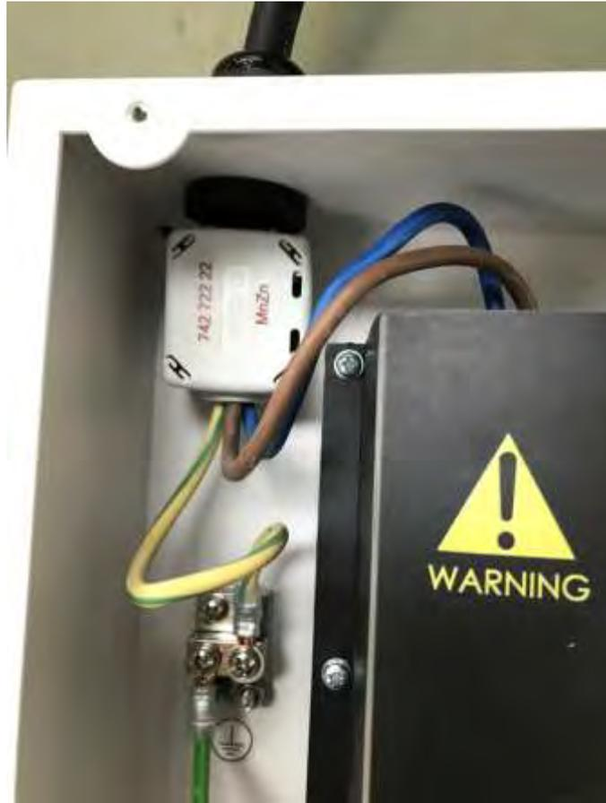
Figure 34: Ferrite installed to AC power cable
