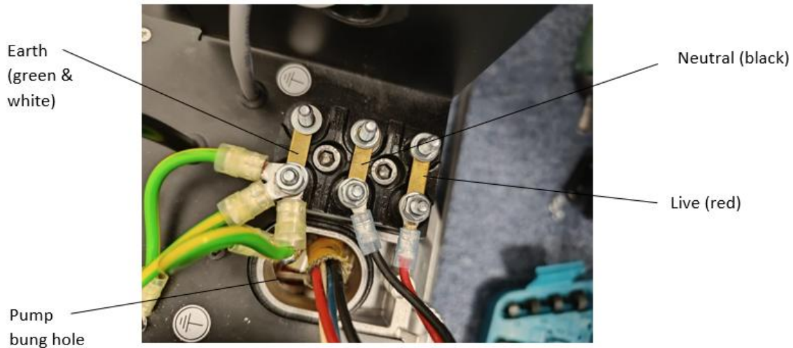
Figure 39: Electrical supply connections
